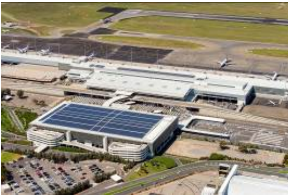
Figure 14: Adelaide Airport 1.17MW Solar Installation
