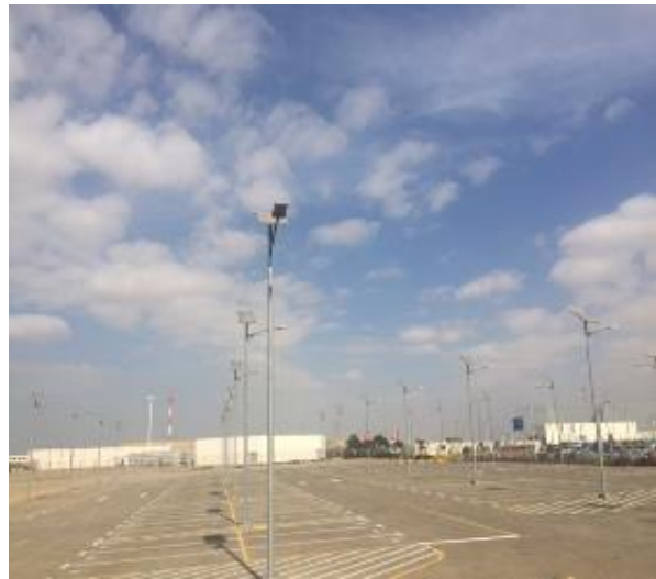
Figure 34: Car parking area of SAA (2)
