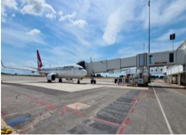
Figure 23: Ground source heat pump in International Terminal Building of Darwin Airport
