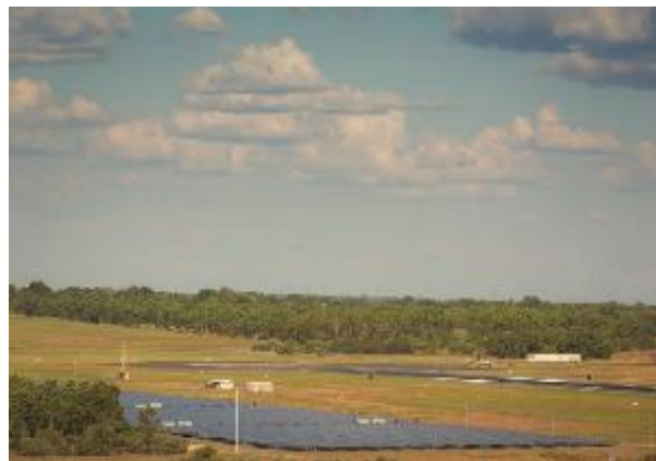
Figure 21: View of Darwin Airport Solar Plant from tower
