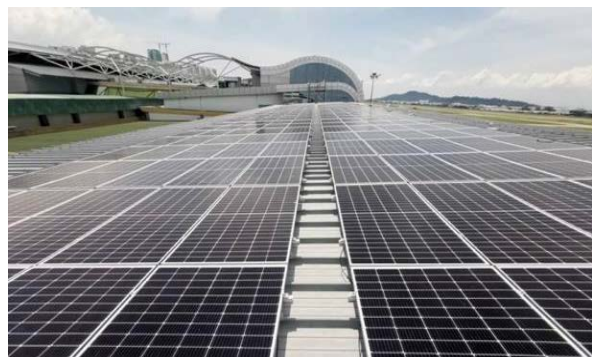
Figure 30: Rooftop, Penang International Airport
