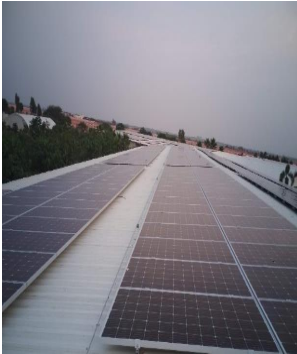
Onsite solar installation (airport office)
