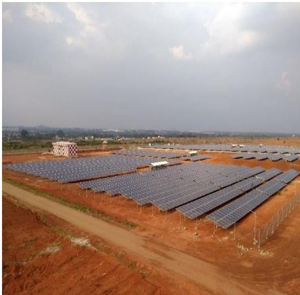
Onsite solar installation (airside ground mounted)
