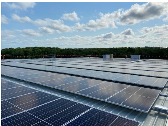
Solar system on cold store Facility 2021
