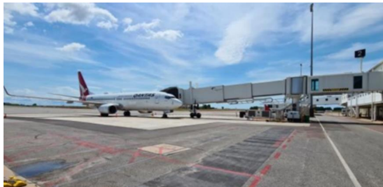
Completion of Bay 2 apron, aerobridge and Pre-conditioned Air December 2021
