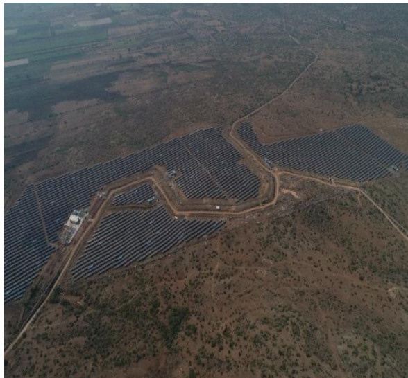
Offsite solar installation
