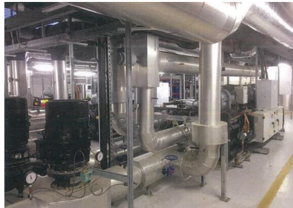
Ground source heat pump in our International Terminal Building
