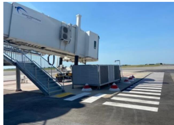
Recently installed preconditioned air unit Bay 2 – November 2021
