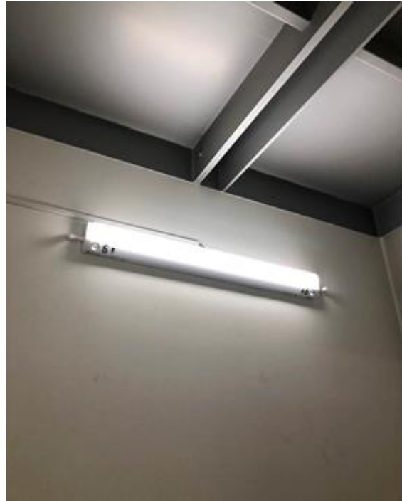
Controlling lighting by installing lightings with motion sensors
