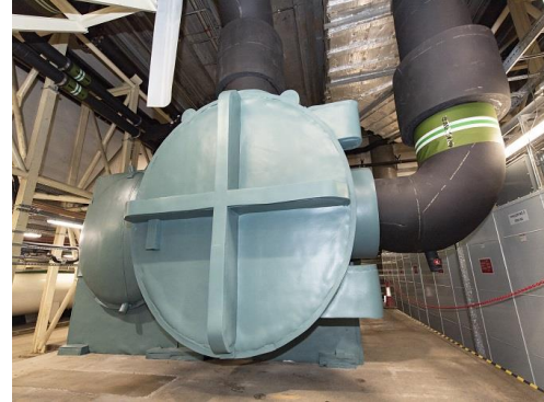
The Weather FACTS is applied in the new energy-efficient chiller system at Terminal 1
