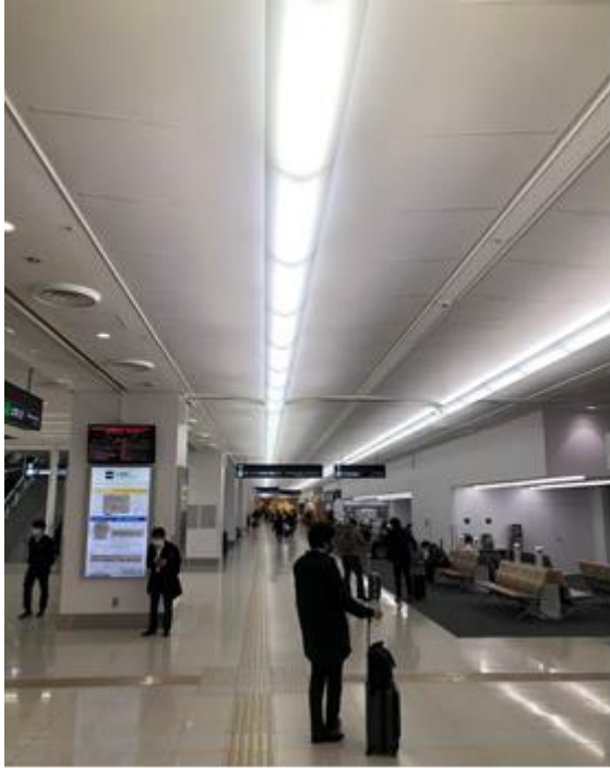
Converting lightings to LED at arrival lobby
