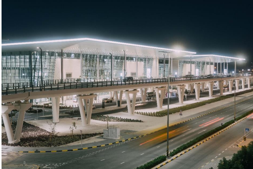
BIA Passenger Terminal Building
