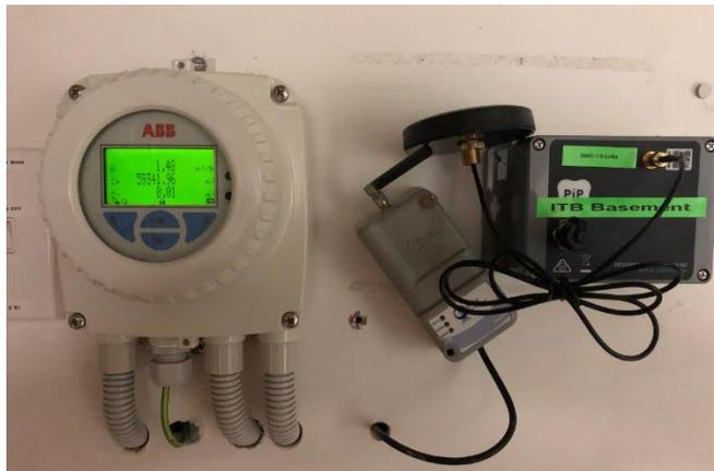
PIP telemetry installed on existing ABB meter
